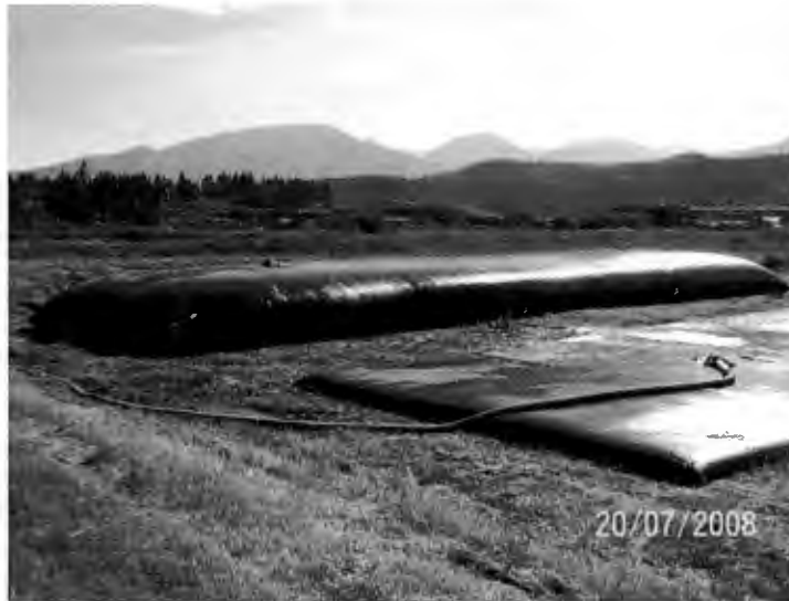
Geotube dewatering tubes. Tubes shown are 60' circumference x 100' long.
